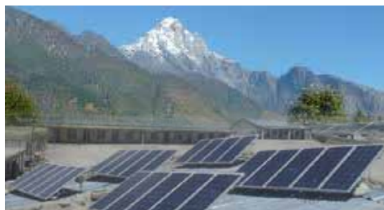
Installed solar system in the districts selected by Renewable Energy Project (REP) funded by European Union
